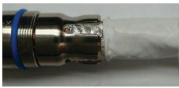
Figure 40: Trimming the outer jacket
