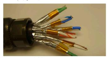
Figure 38: Removing the foil
