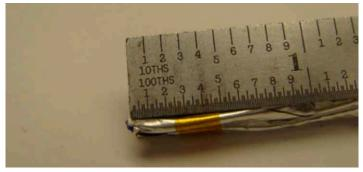
Figure 14: Taping each pair
