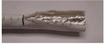
Figure 12: Slitting the cable jacket
