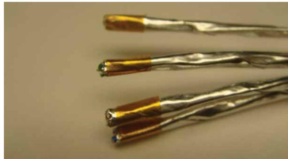
Figure 15: Taping each pair
