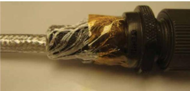
Figure 70: Returning braid to connector
