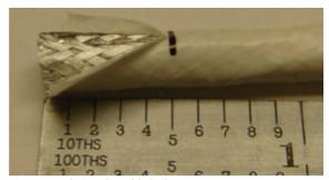
Figure 13: Slitting the cable jacket
